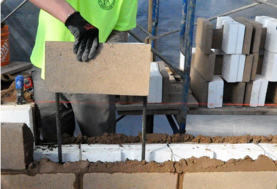
Photo shows typical stock pile the mason pulls CMU from
