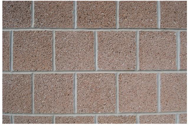
When Split Face and Decro Face are used together they enhance each other. As do the different sizes-16" high  $\times 24$ " long with 4" high  $\times 24$ " long.
