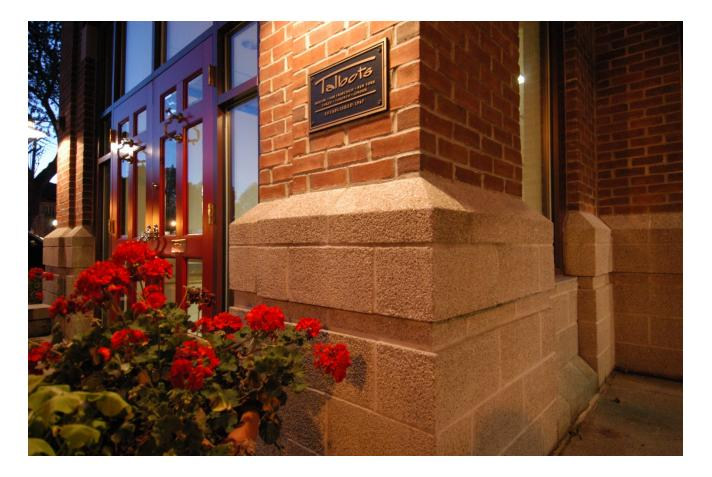
Simple inexpensive details such as single scores in a quarter bond with the scores tooled in. . . . take on an upscale appearance in sand weathered Decro Face.
