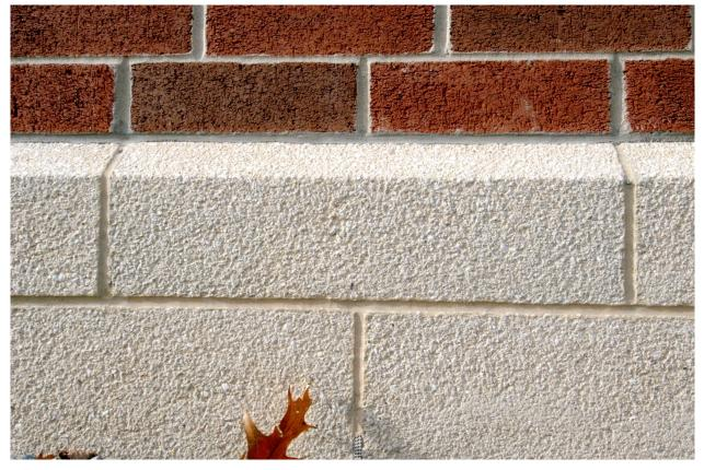
Selected sands that simulate natural limestone make an attractive wall base and rounded watertables for clay. Let us help by providing specification language and details for differential movement between clay and concrete:
