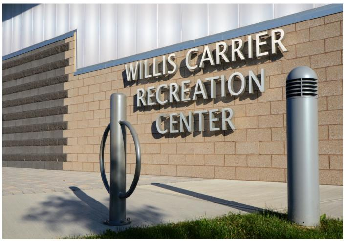
Concrete Masonry makes it easy to design interesting patterns of color and texture. There are no special connections to detail, just indicate on the plans where the masons install each type cmu. Here you see alternate courses of Beamish Artisan Roc <sup>BC</sup> Split Face, and Beamish Ground Face transitioning into Stoney Shore Ground Face.
