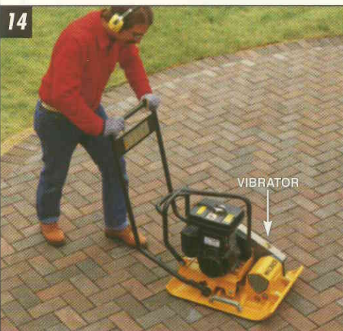
14 TAMP THE PATIO with a flat-plate vibrator after all the pavers are installed. Tamp entire outside edge first, then circle in.
