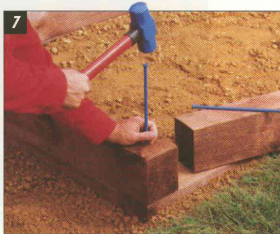
INSTALL LANDSCAPE TIMBERS for edging in areas where you need to change levels or step down. Be certain to overlap corners.
