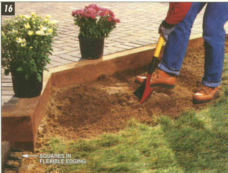
16 LANDSCAPE around the completed patio with flowers, shrubs and grass. Grass will root through the open spaces in flexible edging to anchor it in place.
